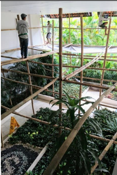
Painting work being audited
